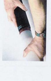
Step 6: Feed fill line and electric ignitor wires through threaded retainer, ensure threads are facing motor case. Tighten retainer all the way, no threads showing.
